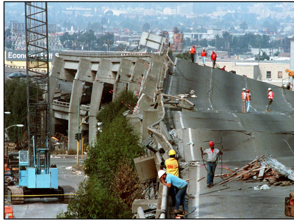
6.9 Loma Prieta Earthquake, 1989
