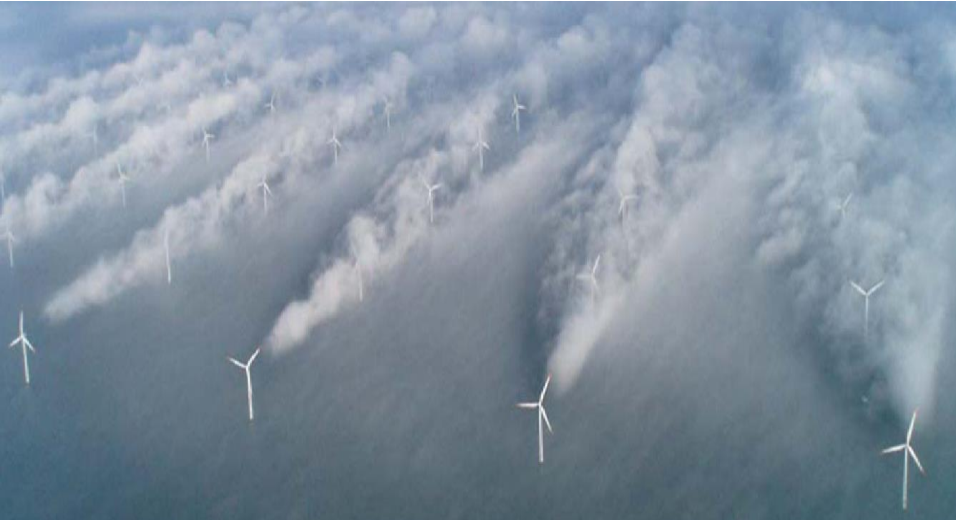
Horns Rev I Offshore Wind Plant
