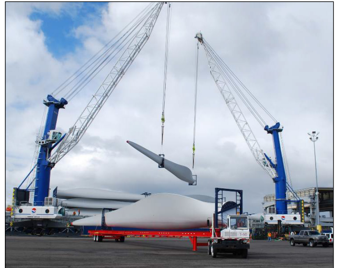
Specialized cranes lifting a wind turbine blade. Photo courtesy of Port of Vancouver USA
