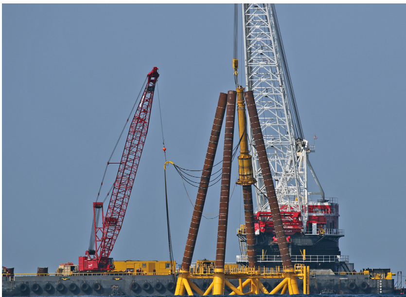
Installing the foundation at Block Island Wind Farm.
