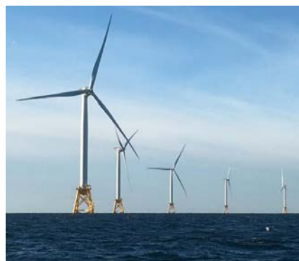
Block Island Wind Farm
