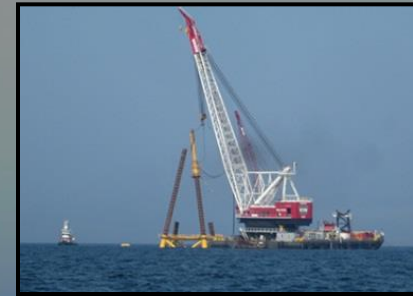
Construction: Drilling and Pile Driving
