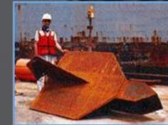
Driven anchor plate (usually vibratory)
