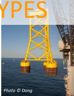
Photo © Dong Suction bucket at DONG BKR01
