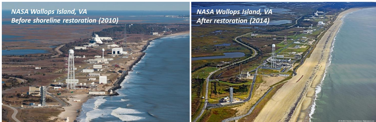
Figure 15. NASA’s Wallops Island Flight Facility, VA before and after restoration using OCS sand.
