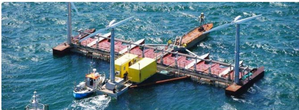
Figure 4. Poseidon 37 (Shown with Wind Turbine Configuration)
