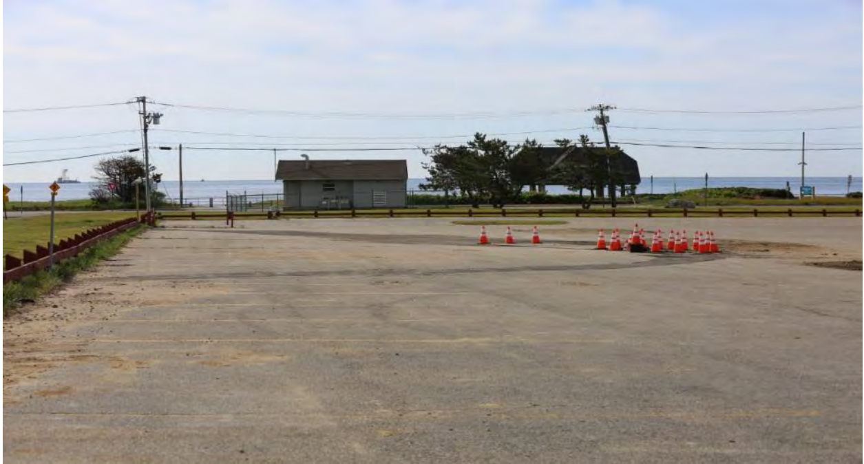
6/11/2016 Scarborough Beach State Park-Photo0293: Onshore work complete at Scarborough Beach State Park. CLB Big Max on horizon laying cable at sea.
