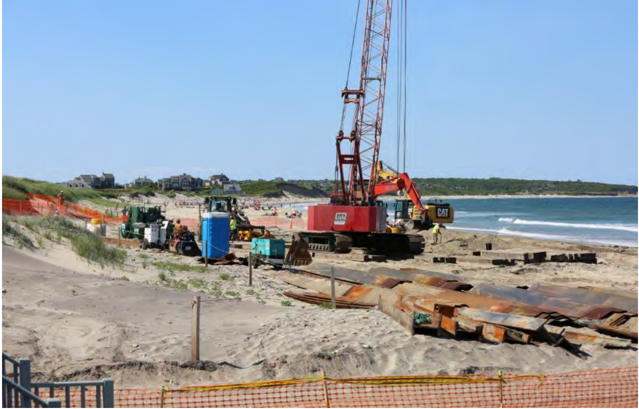
6/26/2016 Block Island Town Beach – Photo 1003: Cofferdam removed and backfilling excavated sand.
