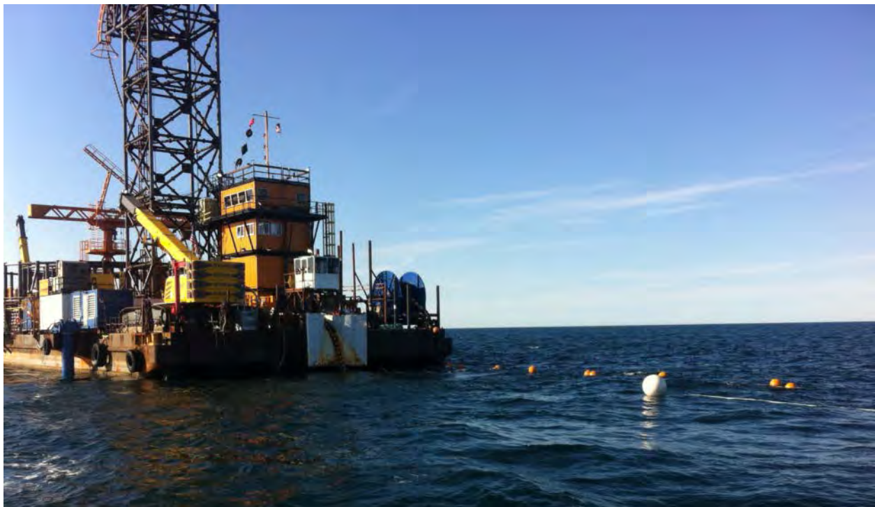
Figure 6. Marker buoys from the jet plow rigging showing the approximate location of the plow on the seabed
