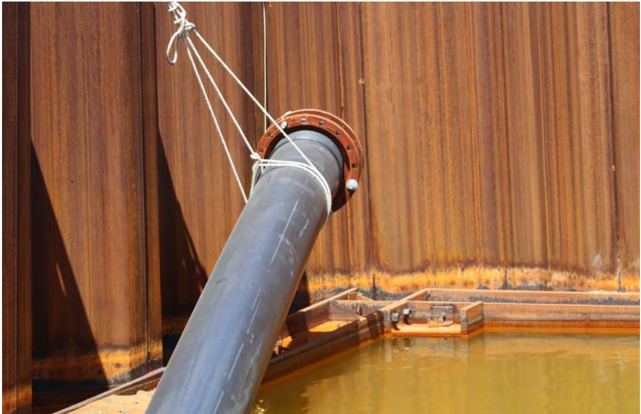
6/15/2016 Block Island Town Beach – Photo 3164: Interior of cofferdam, BITS cable conduit.
