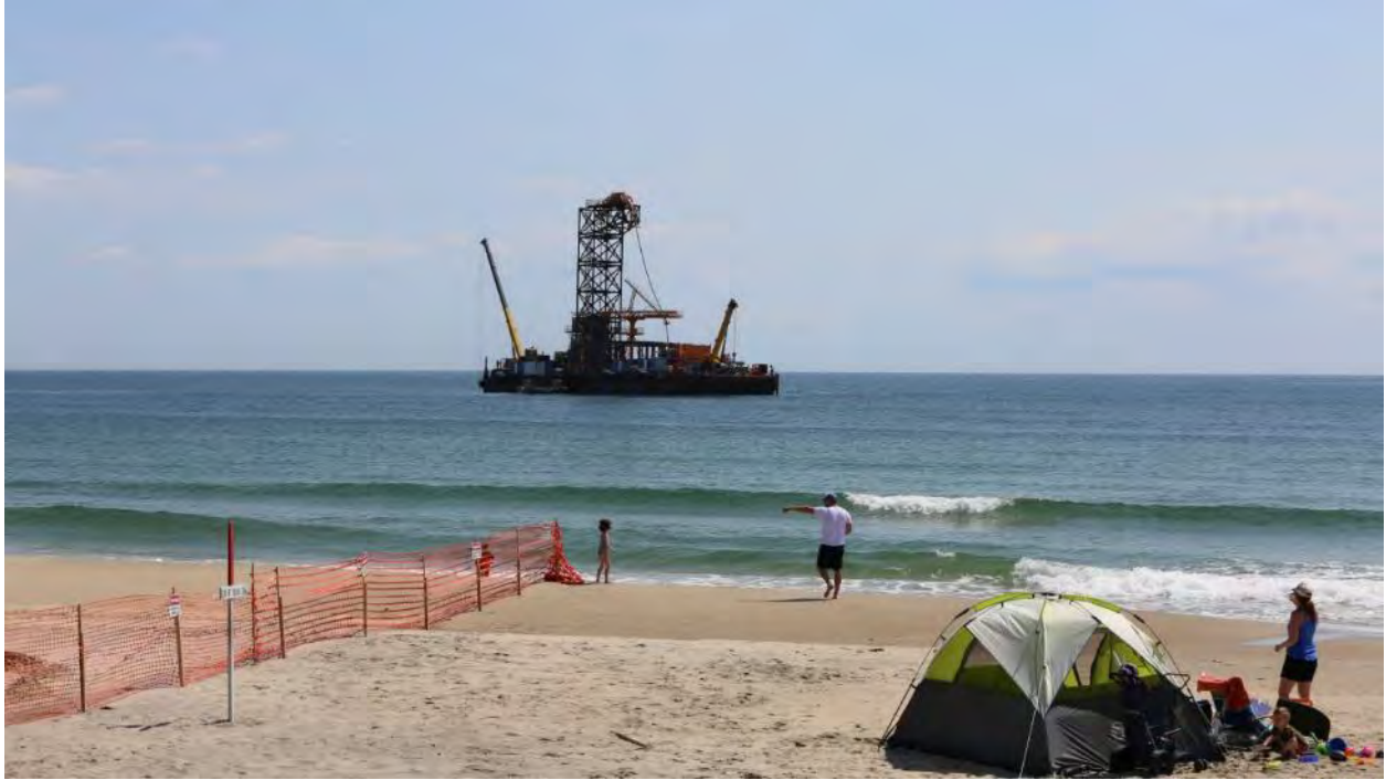
6/22/2016 Block Island Town Beach – Photo 04650: CLB Big Max anchored off Crescent Beach preparing for land sea transition of BITS cable.
