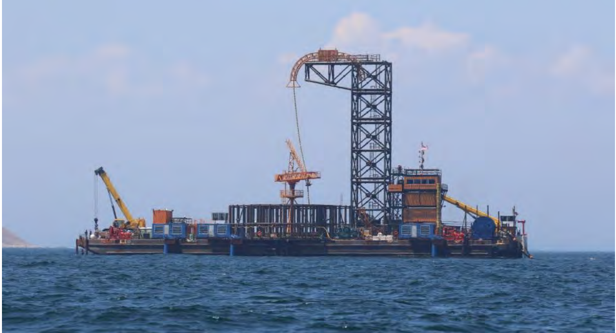
Figure 3. Cable Lay Barge CLB Big Max
