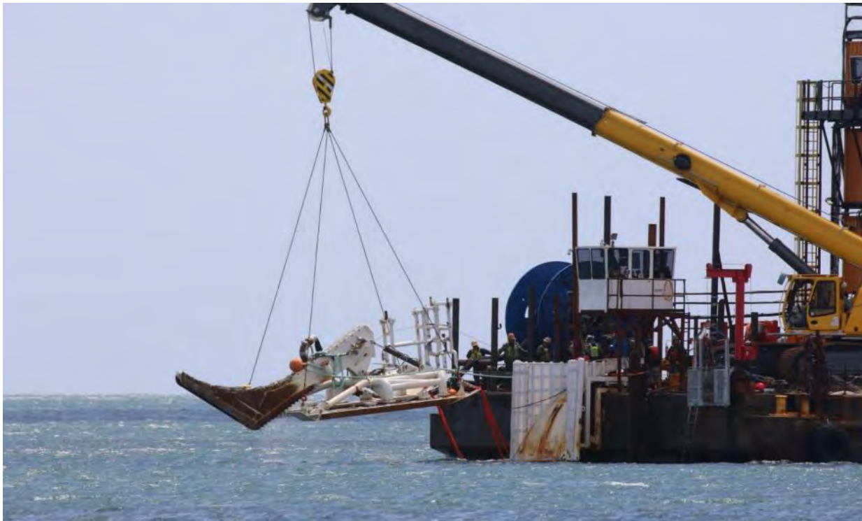
Figure 4. Jet Plow being lowered into water
