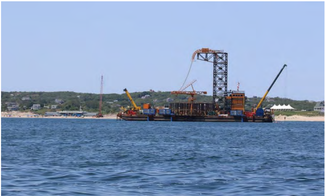
6/22/2016 Offshore – Photo 3560: CLB Big Max anchored off Crescent Beach preparing for land sea transition of BITS cable. Fredrick J. Benson Pavilion at Town Beach in background.
