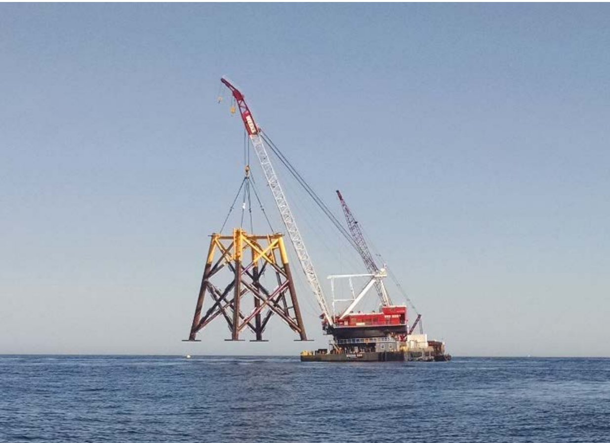
US EAST COAST DERRICK BARGE SETTING JACKET
