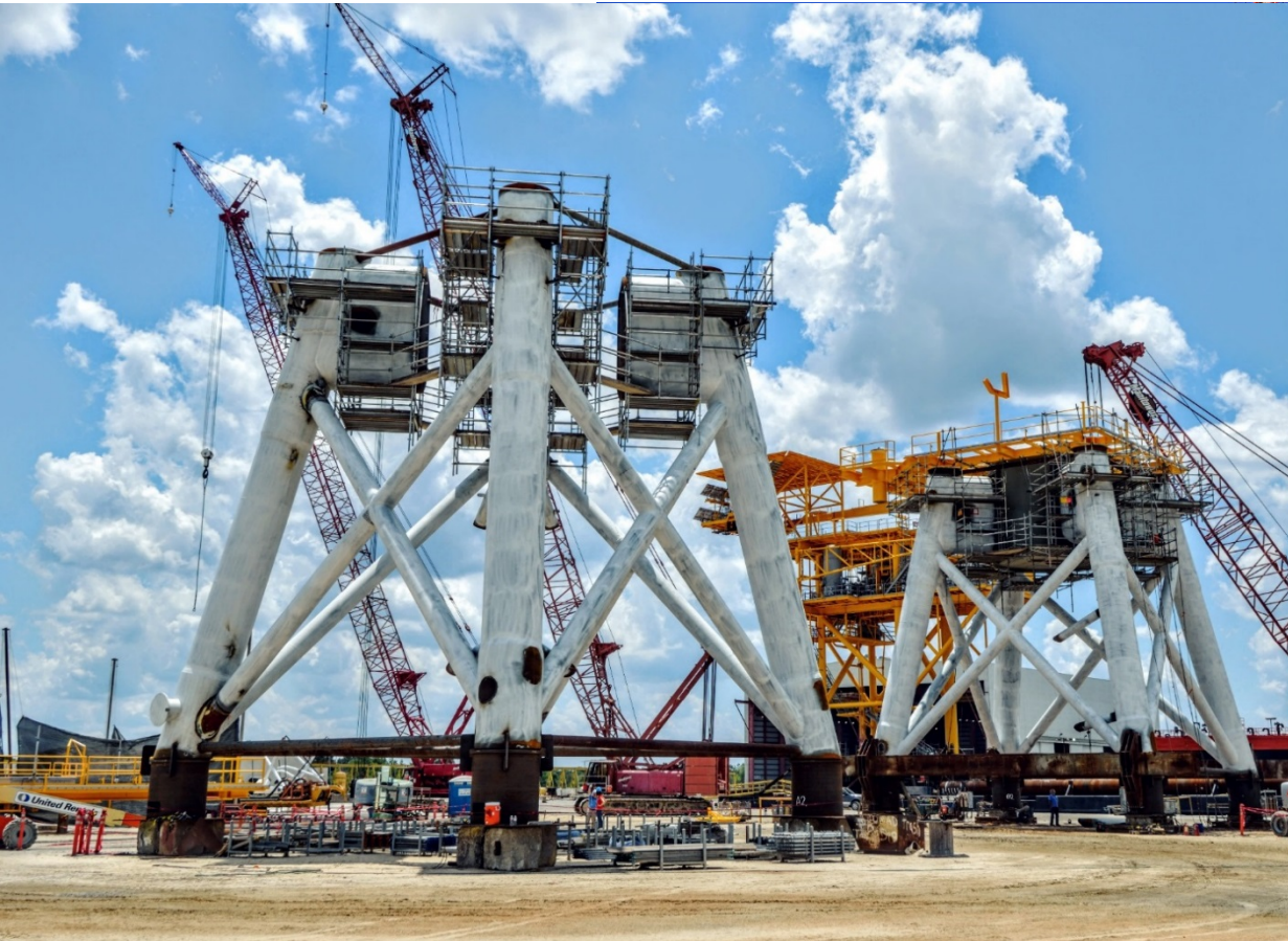
ASSEMBLING TRANSITION DECKS
