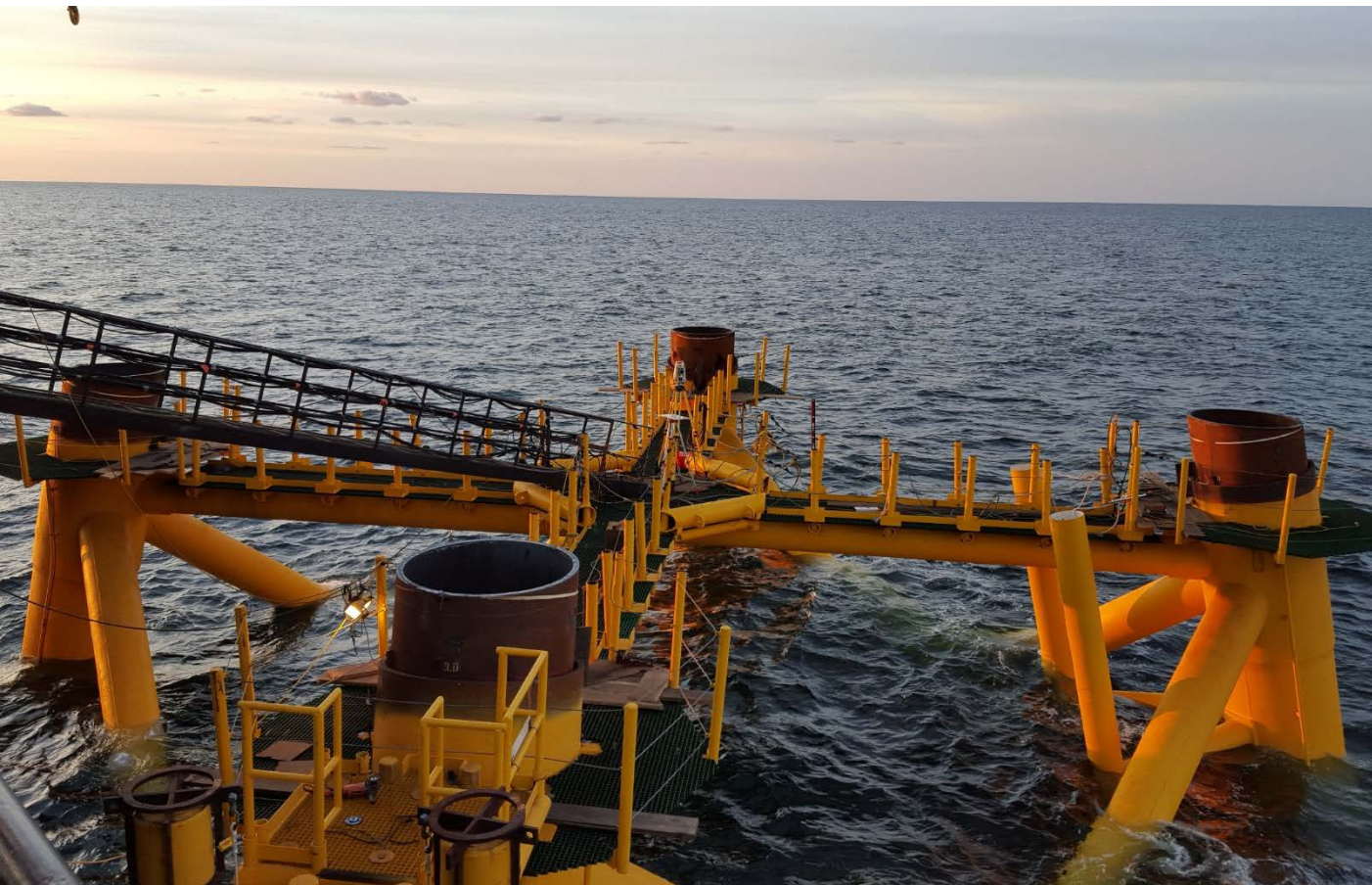
CUTTING PILES OFF LEVEL
