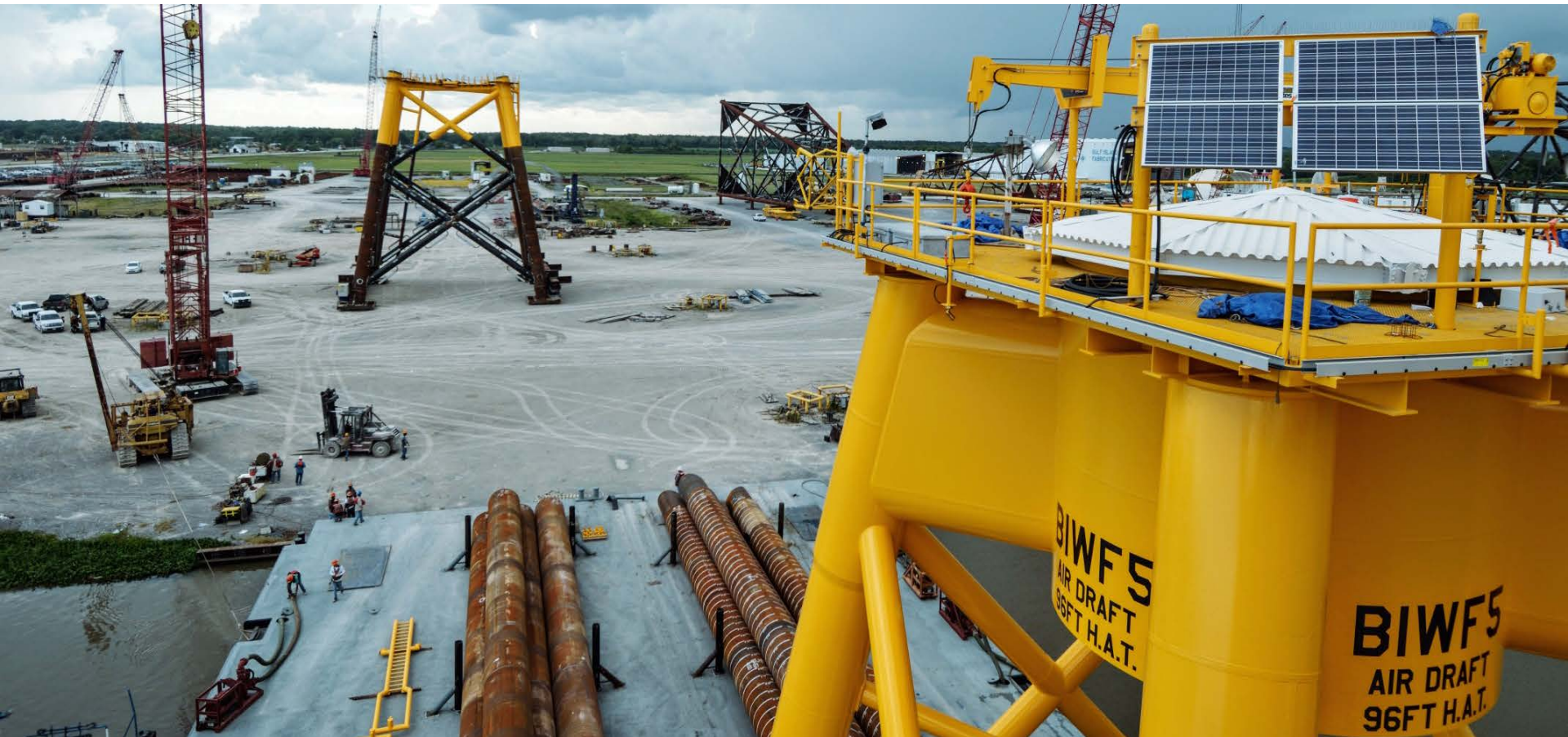
SEAFASTENING TRANSITION DECKS AND PILES ON US CARGO BARGE
