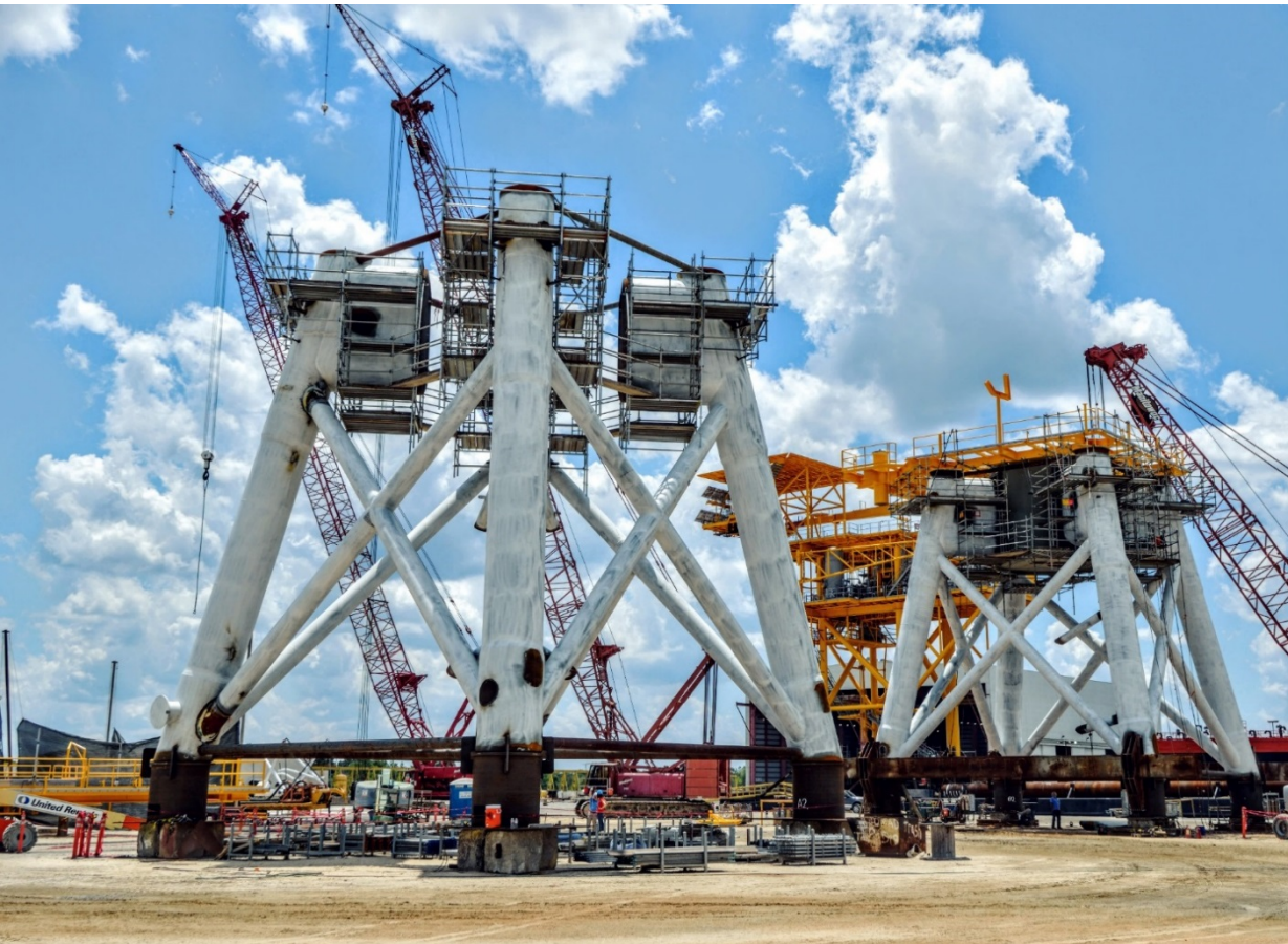
ASSEMBLING TRANSITION DECKS
