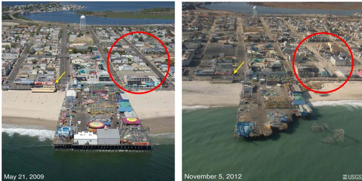
Figure 15. Before and after Hurricane Sandy storm damages (Seaside Heights, New Jersey).
