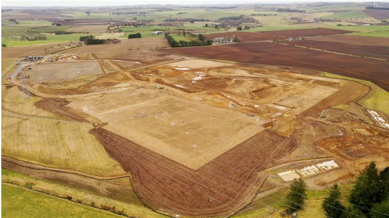
Figure 3: Moray East Substation Site - March 2019
