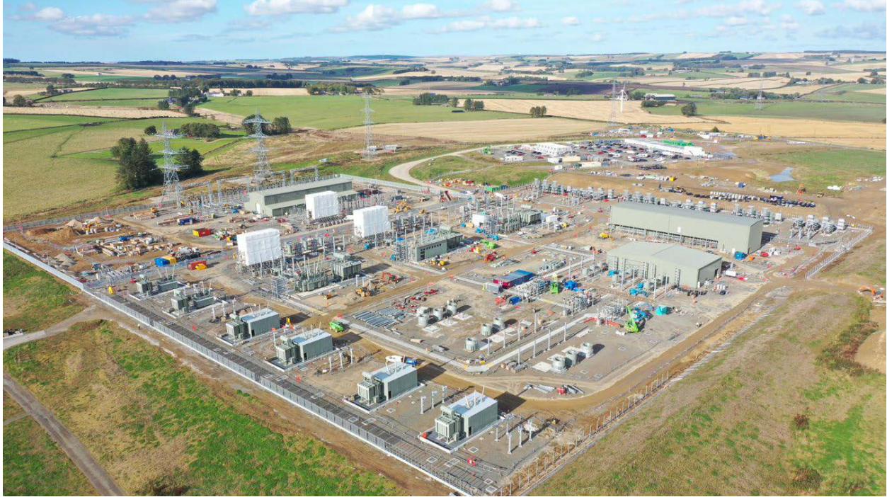
Figure 4: Moray East Substation Site - February 2020
