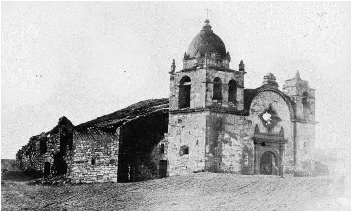
Figure 49. Mission San Carlos Borromeo de Carmelo Church, 1793–1797, Carmel, California (National Register # 66000214). One of the earliest California Spanish Missions. Photographed in 1860 and subsequently restored beginning in the 1920s (From Library of Congress 2013b).
