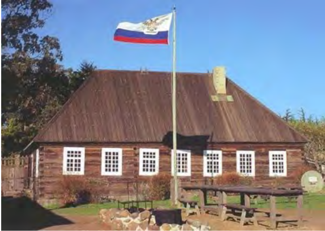
Figure 29. Rotchev House, ca. 1836, Fort Ross Historic District, Jenner, California (National Register # 66000239). This heavy timber-frame vernacular home is a rare example of a building associated with early European settlement in California (From Roundtree and Xie 2011).
