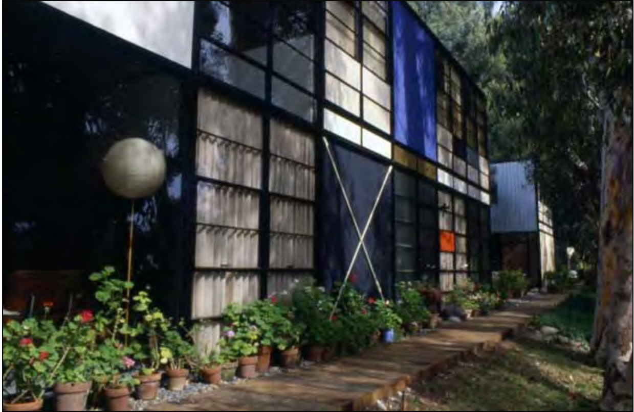
Figure 39. Eames House, 1949, Pacific Palisades, California. Moderately scaled International-style house designed by master architects Charles Eames and Eero Saarinen (National Register # 06000978). Image courtesy of Eames Office (© 2013 Eames Office, LLC, eamesoffice.com ).
