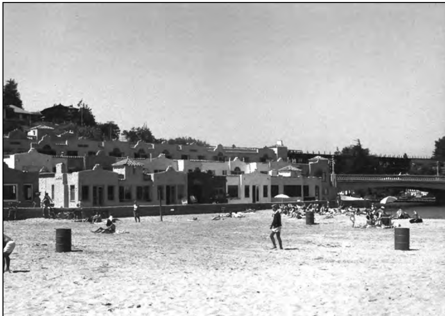
Figure 35. Venetian Court Apartments, 1925, Capitola, California (National Register # 87000574). An example of the Spanish Colonial Revival style adopted for multiple-family residences. Photographed in 1986 (From National Park Service 1987a).
