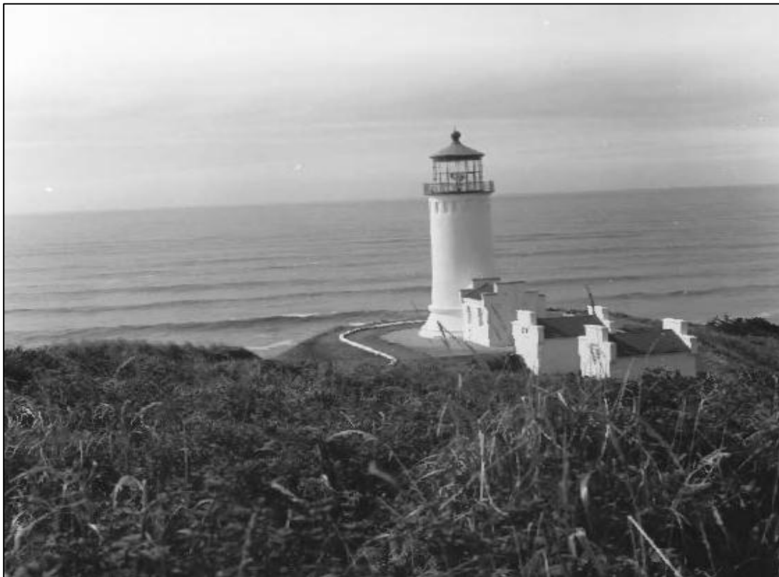
Figure 54. North Head Lighthouse, 1898, Cape Disappointment Historic District, Ilwaco, Washington (National Register # 75001864). The second of two lighthouses constructed at Cape Disappointment, the North Head Lighthouse served as an aid to navigation at the cape's northwestern spur. It features one observation deck and an attached keeper's quarters. Photographed in 1971 (From National Park Service 1975).
