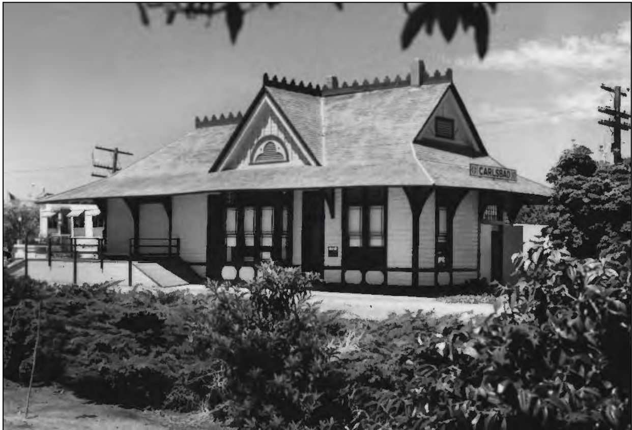
Figure 66. Carlsbad Santa Fe Depot, 1887, Carlsbad, California (National Register # 93001016). Atchison, Topeka and Santa Fe Railway (Santa Fe) architect Fred R. Perris designed this Folk Victorian–style train depot. Photographed in 1992 (From National Park Service 1993).
