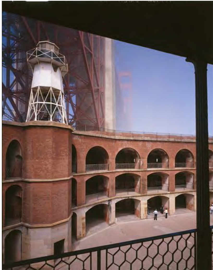
Figure 52. Fort Point 1861, San Francisco, California (National Register # 70000146). A masonry fortress, this National Historic Site features a courtyard surrounded by three stories of tiered brick arches and an octagonal metal lighthouse capping the northwest tower (From Library of Congress 2013c).
