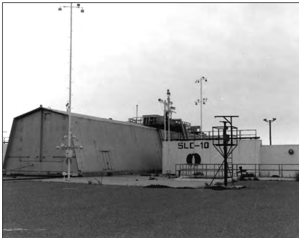
Figure 53. Space Launch Complex 10, 1958, Lompoc, California (National Historic Landmark # 86003511). One of two launch pads built by the Douglas Aircraft Company to support combat training launches. Space Launch Complex 10 consists of a Blockhouse, two concrete launch pads, a prefabricated launch shed, and some support equipment. Photographed ca. 1986 (From National Park Service 1986b).
