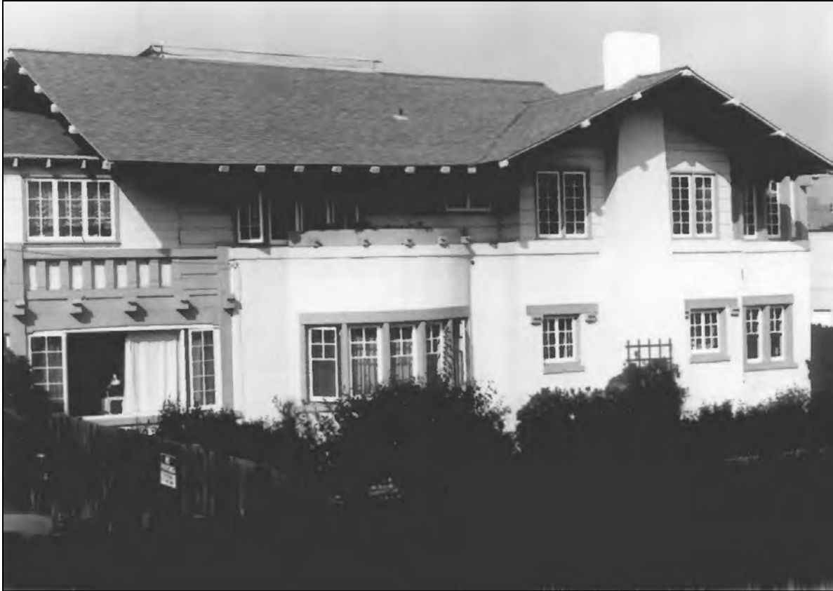
Figure 37. Warren Wilson Beach House, 1911, Venice, California (National Register # 86001666). A grand Craftsman-style residence. Photographed in 1975 (From National Park Service 1986a).
