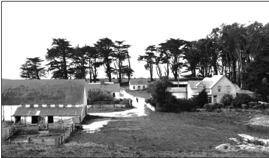
Figure 48. Pierce Dairy Ranch, 1856–1935, Point Reyes National Seashore, near Inverness, California (National Register # 85003324). Large coastal dairy ranch established in 1856 that includes vernacular residences, dairy houses, barns, and a school house. Photographed in 1980 (From National Park Service 1985).
