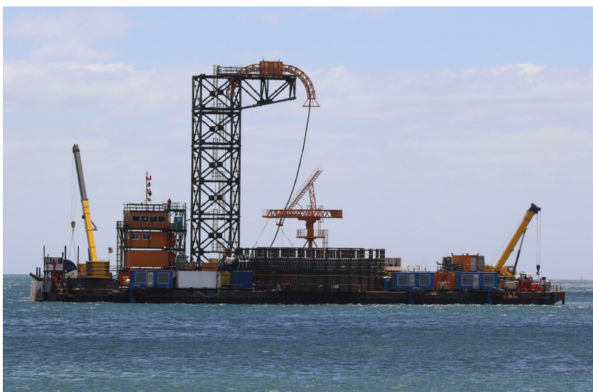
Cable Lay Barge CLB Big Max.
