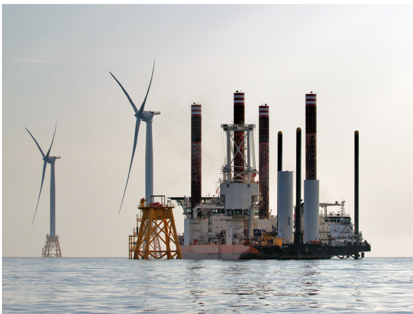
Installing wind turbines at Block Island Wind Farm.
