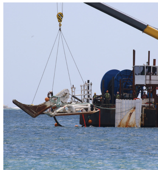
Dredge used for cable laying.
