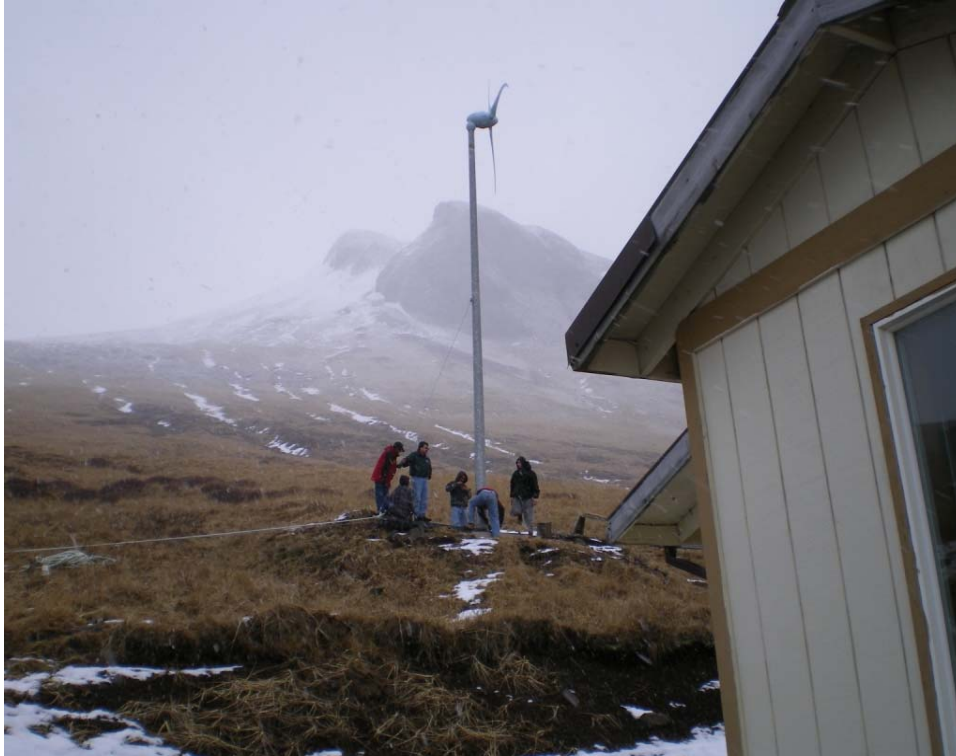
Figure 148. Wind turbine being erected in Akutan, February 2010. Photo by Crystal Callahan.
