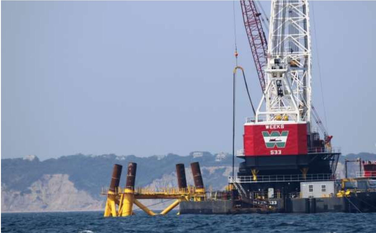
**Figure B-15.9/02/2015 Offshore Photo 1010: WTG 3 with first set of piles driven by Weeks Derrick Barge 533. Block Island in the background.**
