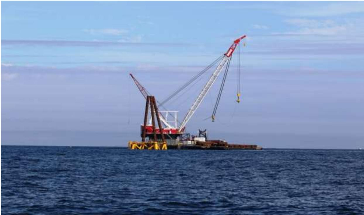
**Figure B-10. 8/23/2015 Offshore Photo 0186: Weeks Barge 533 just placed third pile at WTG 3.**
