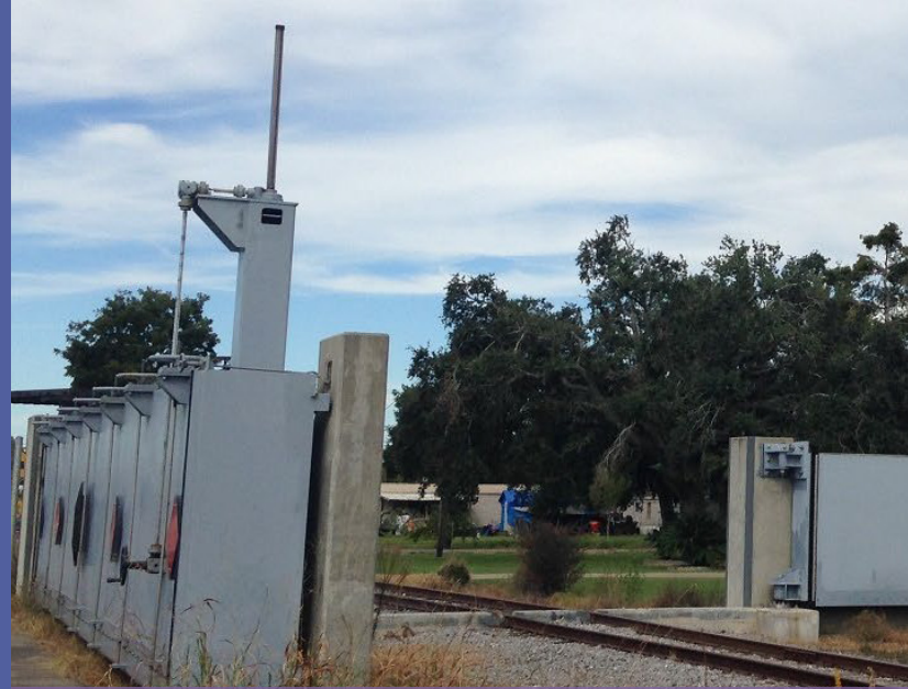
Floodwall in Plaquemines Parish, Louisiana
