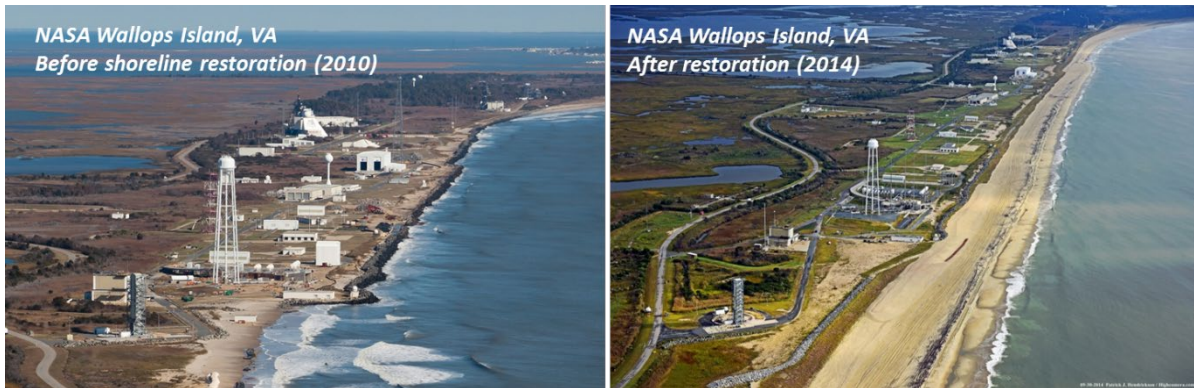
Figure 3. NASA's Wallops Island Flight Facility before and after restoration
