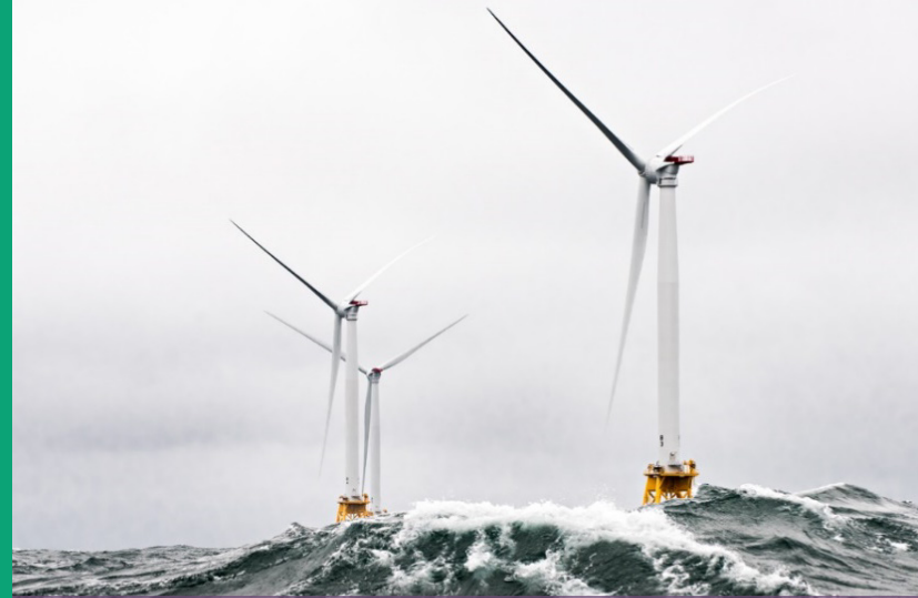
Block Island Wind Farm with jacket-type substructures (yellow)
