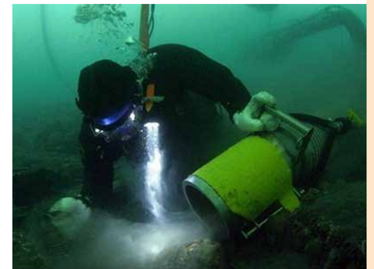
Small suction dredge operated by a diver. Image courtesy of Diver's World Antzoulis, 2017.
