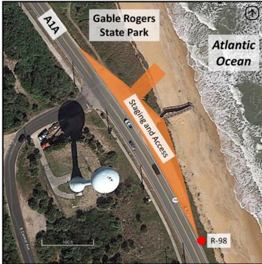
Photo 1a. Staging and access area near the beach access at Gamble Rogers SRA at R-98.
