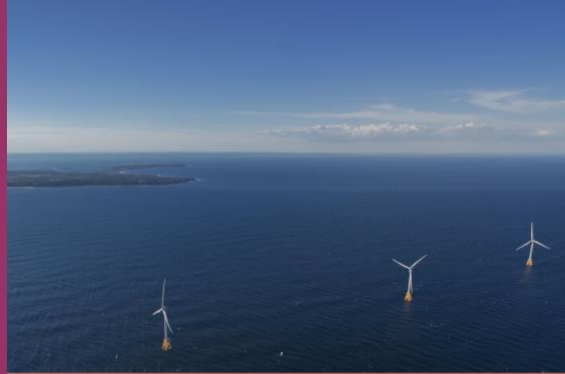
Block Island Wind Farm, the first operational offshore wind energy facility in North America, located ~5 km (3 miles) off the southeast corner of Block Island
