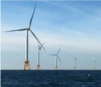
Block Island Wind Farm offshore Rhode Island
