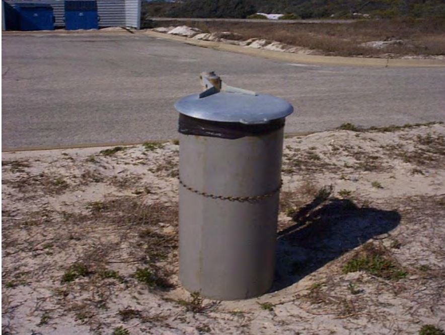
Example of predator proof trash receptacle at Gulf Islands National Seashore. Lid must be tight fitting and made of material heavy enough to stop animals such as raccoons.
