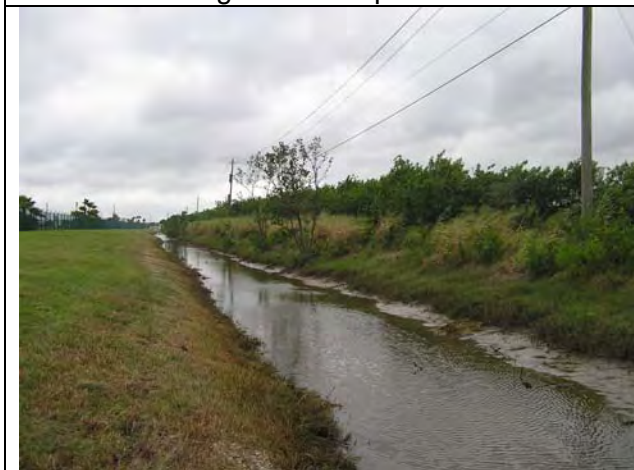
3. W-1: South conveyance ditch, facing east.
