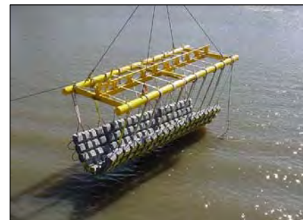
Figure 7 Concrete Mattress on Deployment Frame
