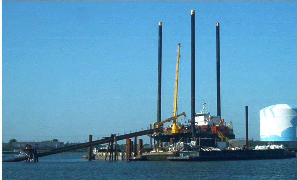
Figure 3 HDD Entry Side Operations from a 200 Class Lift Boat
