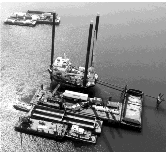
Figure 1 - Typical HDD Marine Spread
