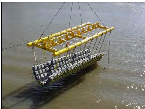
Figure 3-9 Concrete Mattress on Deployment Frame
