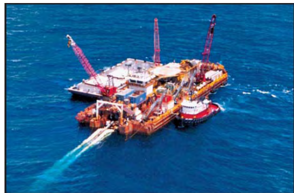
Figure 3-1 Typical Pipelay, Plowing, and Backfill Spread (courtesy of Horizon Offshore)
