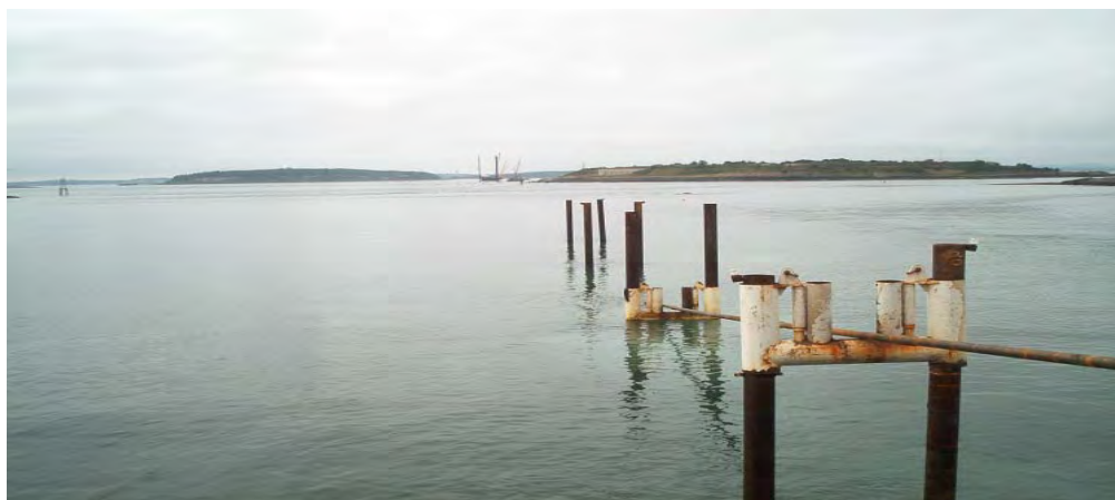
Figure 4 HDD Exit Side Operation – Riser Structure
