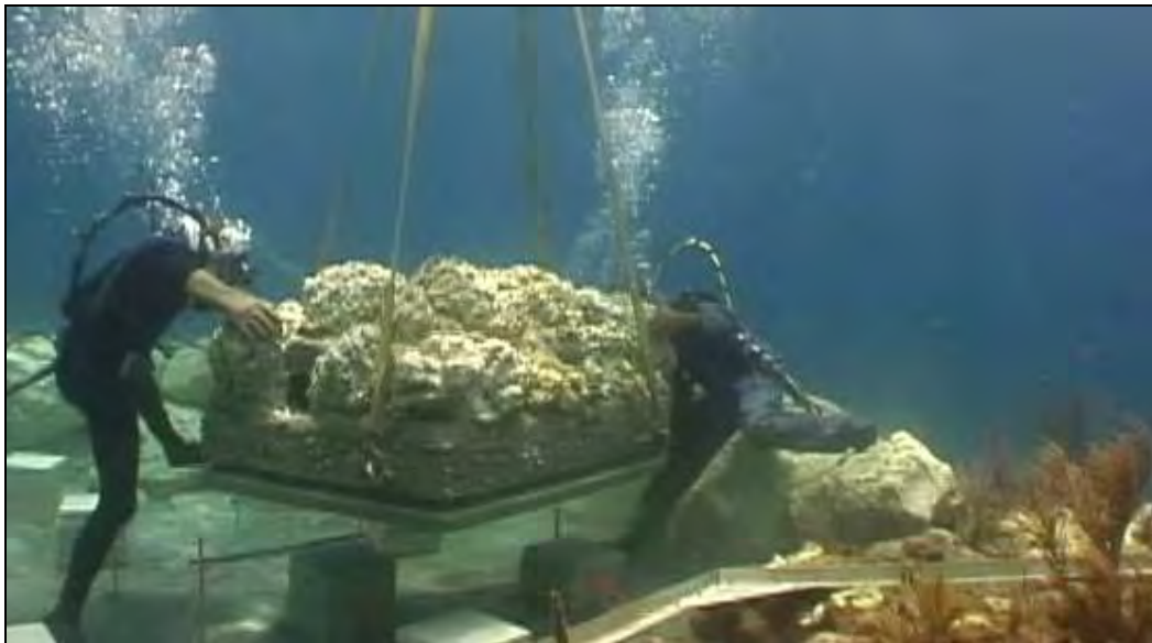
Figure 15 Habitat Replacement Module Deployment Requiring Commercial Dive Operations and Marine Operation Heavy Equipment
