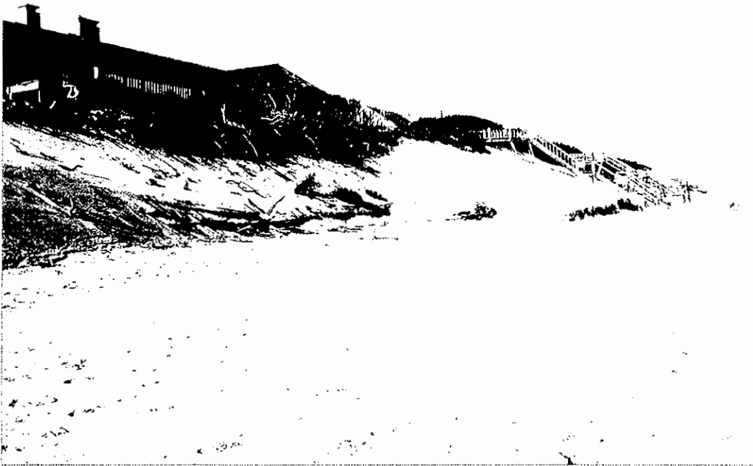
FIGURE 3.17. Bulldozed beach and dune in Indian Beach (recently bulldozed dune in background, dune scraped last season in foreground). Photo taken May 11, 2001, 5:30 p.m.
