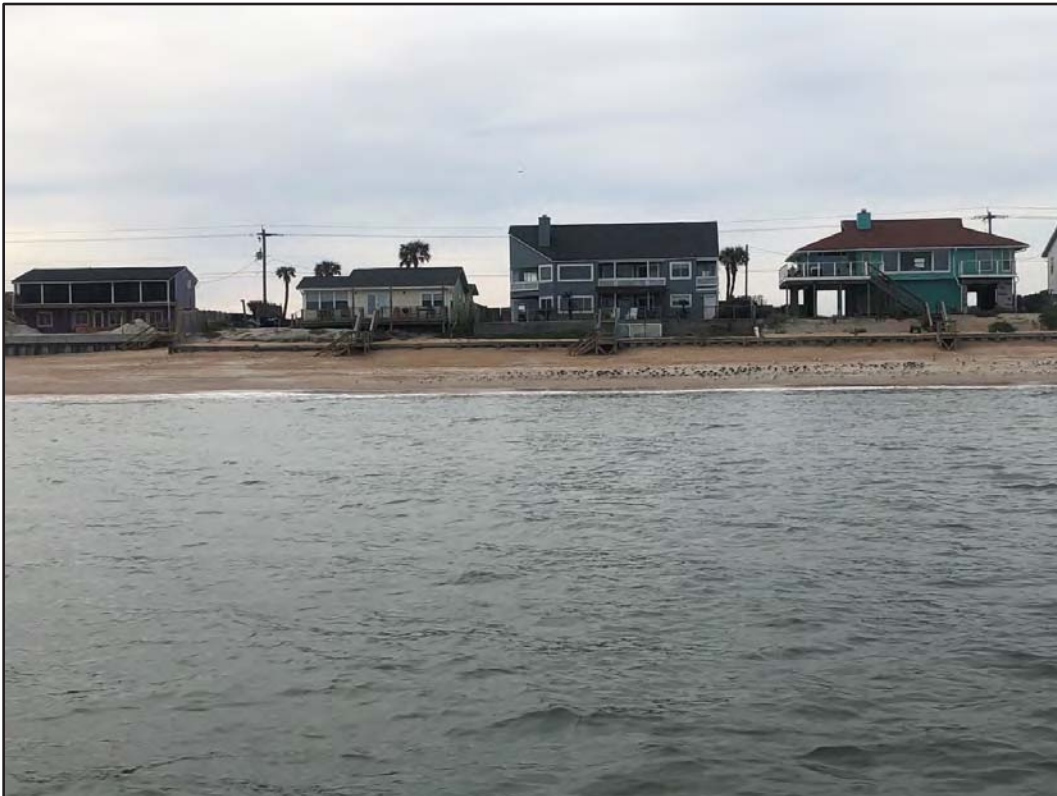
Figure 3-02. Project Area closest line to shore; facing west. Beach homes in the background.
