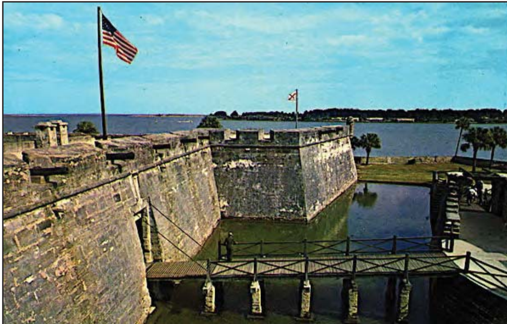
Figure 2-05. Immediately southwest of the inshore Project Area lays the Castillo de San Marcos National Monument (courtesy of the State Library and Archives of Florida).
