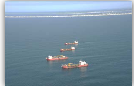
Multiple dredges working off Long Beach Island, NJ
