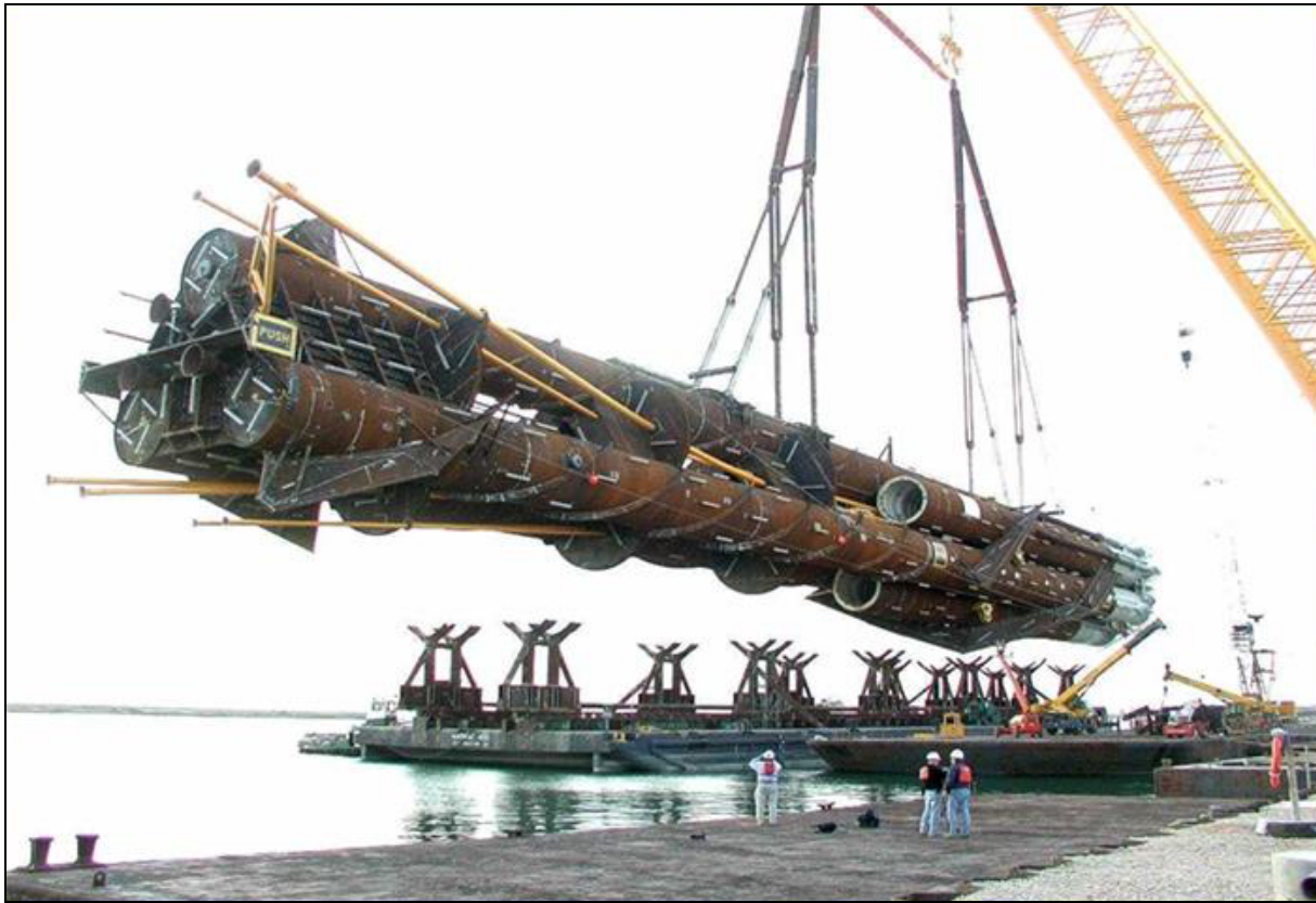
Figure 12. Cylinders of Red Hawk cell spar (photo courtesy of Kerr-McGee).
