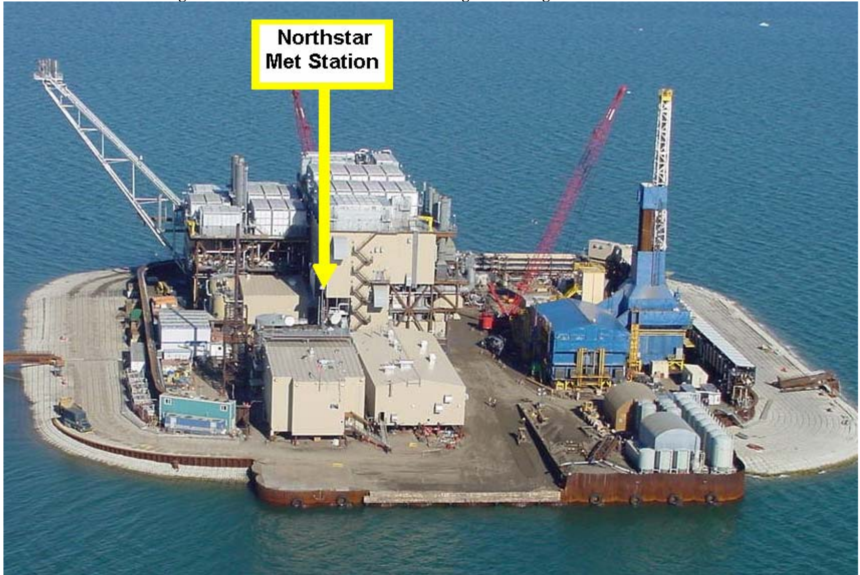
Figure 5-1 Aerial View of Northstar Showing Meteorological Station Location
