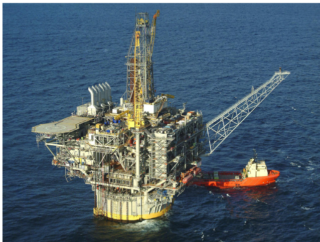
Figure 40. Three development systems: a TLP installed at Magnolia field, a semisubmersible at Thunder Horse field, and a truss spar installed at Holstein field (images courtesy of ConocoPhillips and BP/Marc Morrison).
