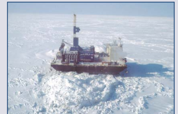
Concrete Island Drilling Station (CIDS)
