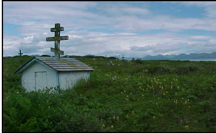
Traditional Structure in the Village of Akhiok, Summer 2005
