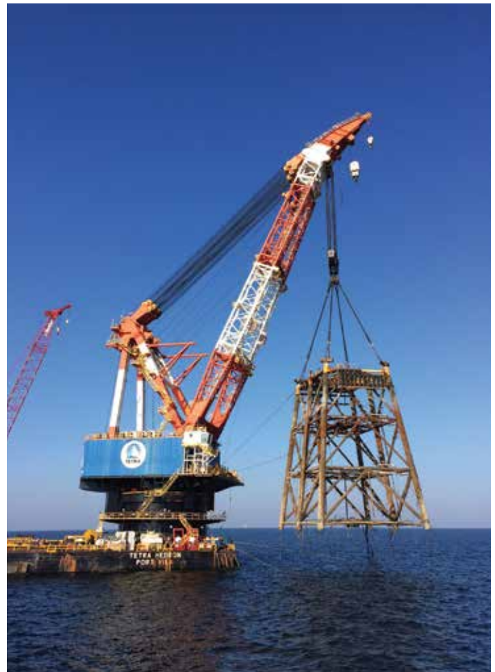
Decommissioning a platform. Photo by Tre Glenn, BOEM.
