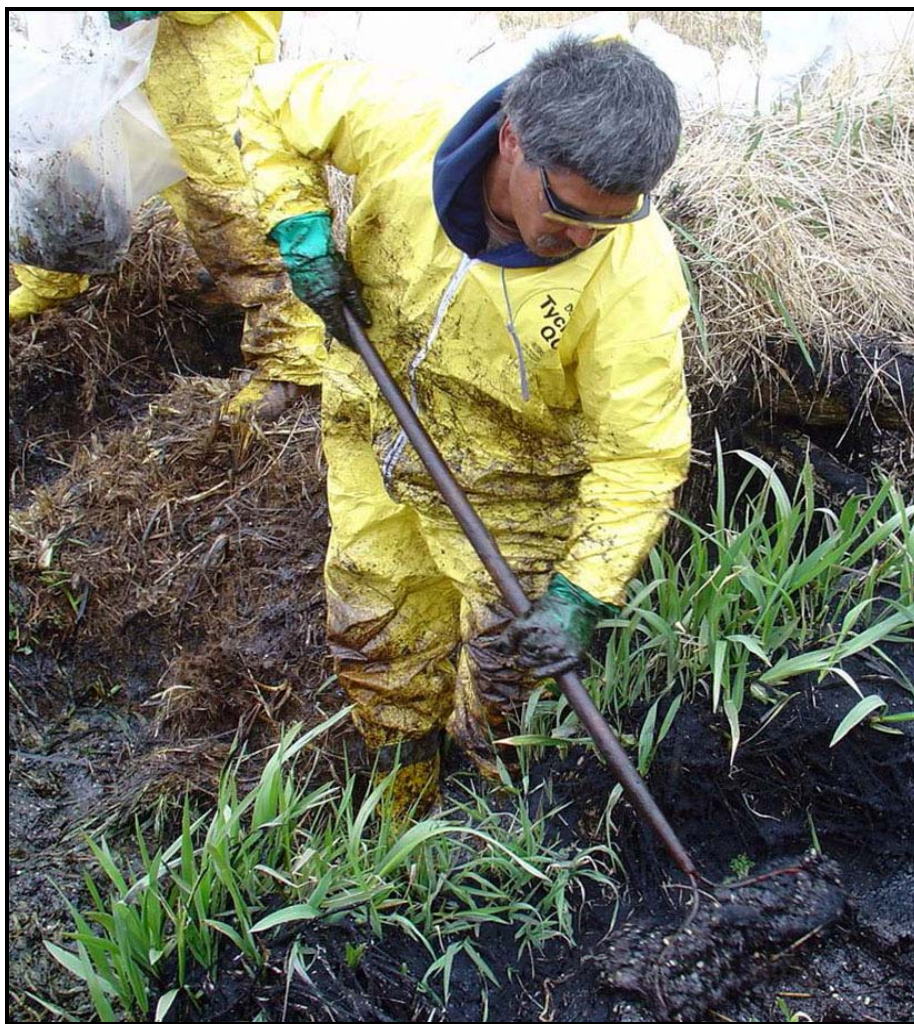
Figure 8. Manual Tilling of Affected Soil near Wreck Site, Winter 2005 Photo Courtesy of U.S. Coast Guard
