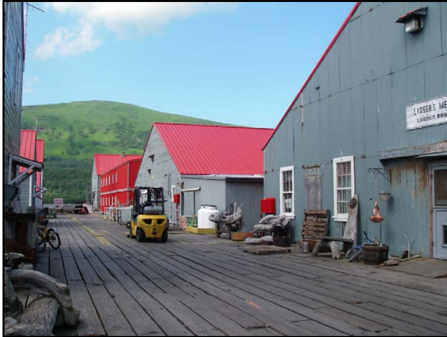
Figure 6-13 Cannery Dock and Store at Larsen Bay
