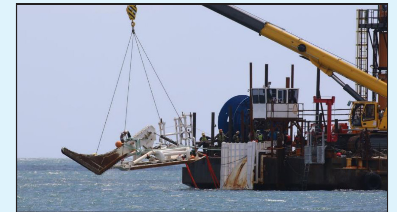
Jet plow being lowered.
