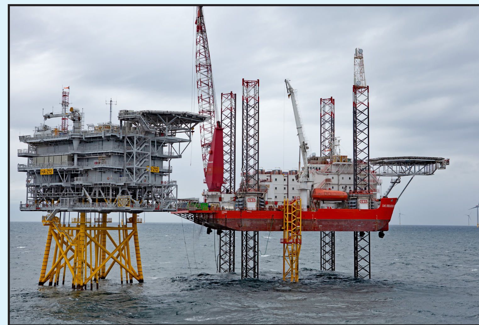
Installation of offshore substation.
