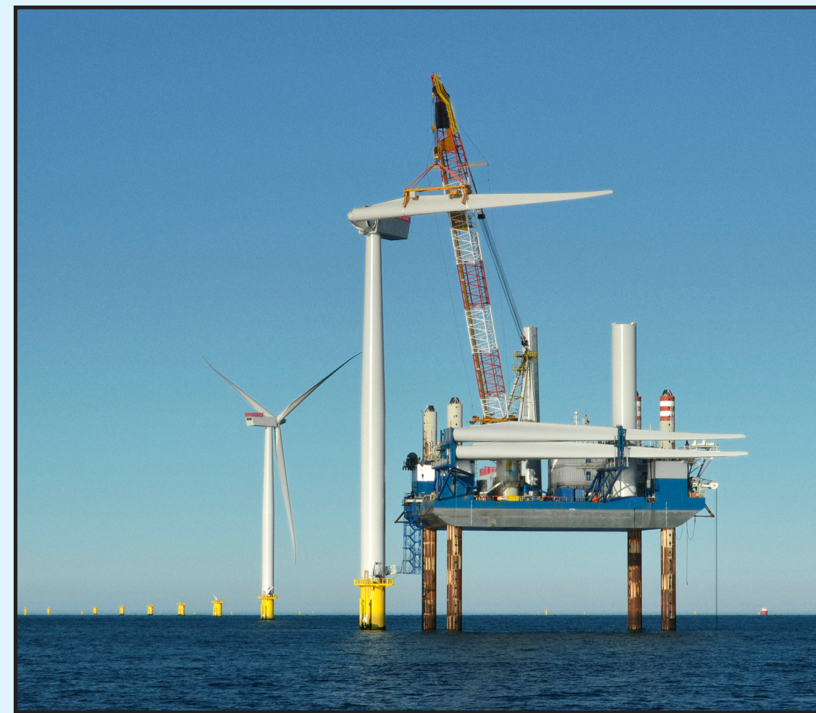
Wind turbine installation.
