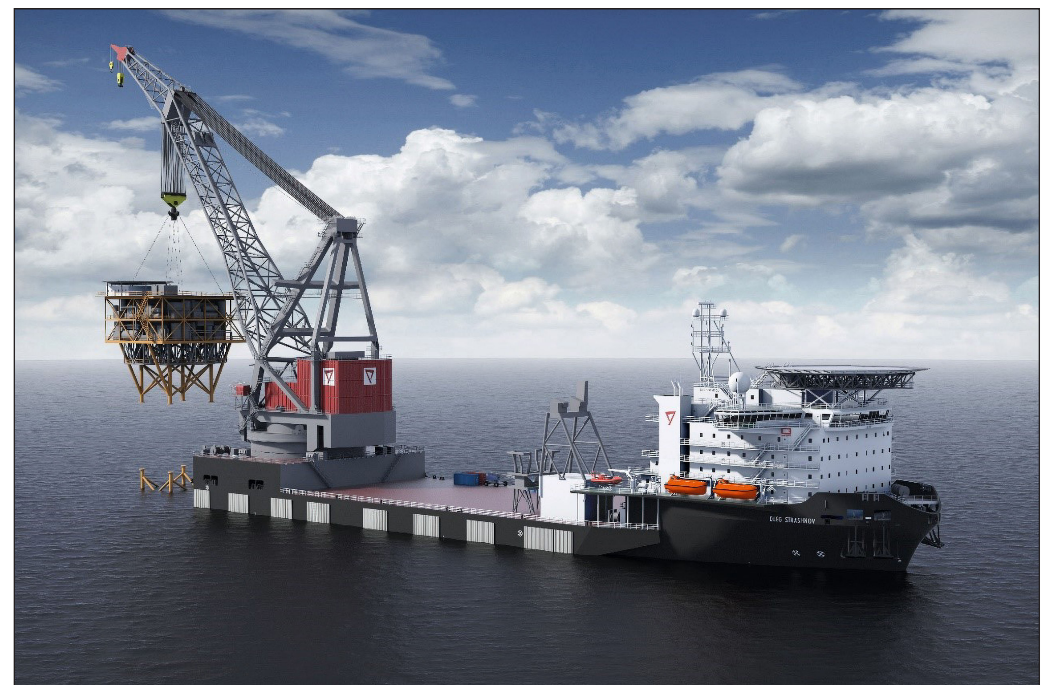
Heavy Lift Vessel Installing an Offshore Substation Platform (Source: DNV 2019)
