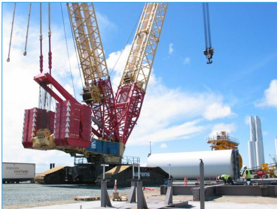
Figure 6.1.2-4. Upending of tower section in load-out port.
