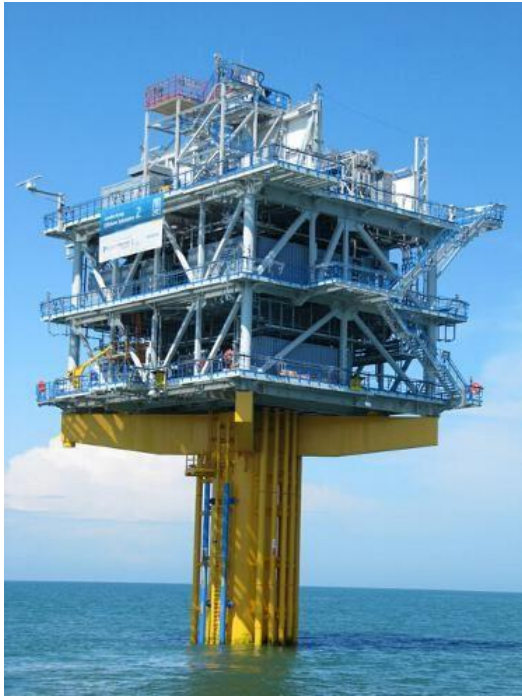
Figure 6.1.1-5. Indicative monopile foundation offshore substation (London Array).
