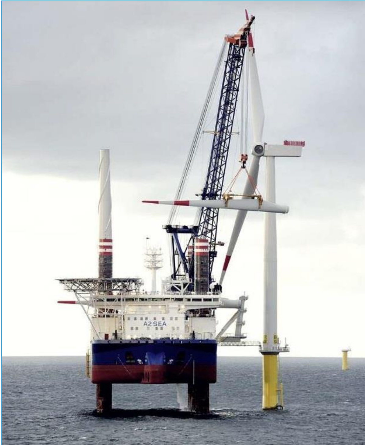
Figure 6.1.2-10. Installation of a WTG blade.
