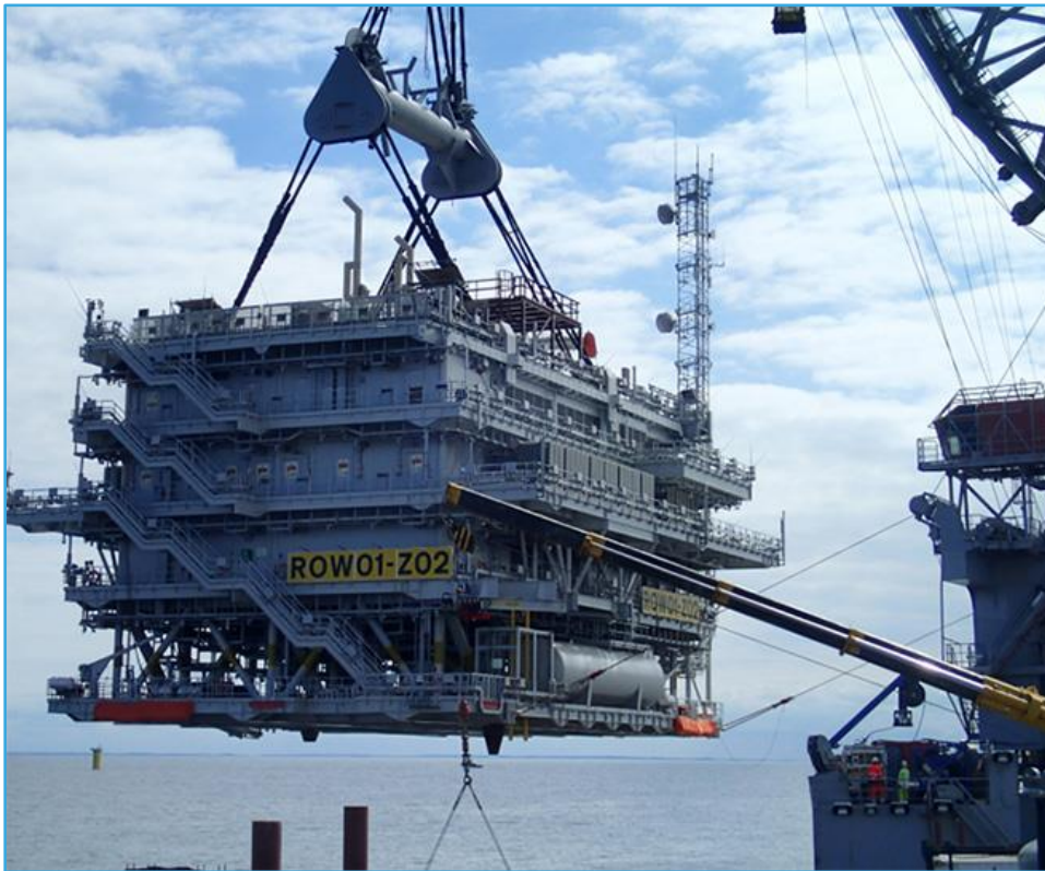
Figure 6.1.2-12. Installation of an offshore substation.
