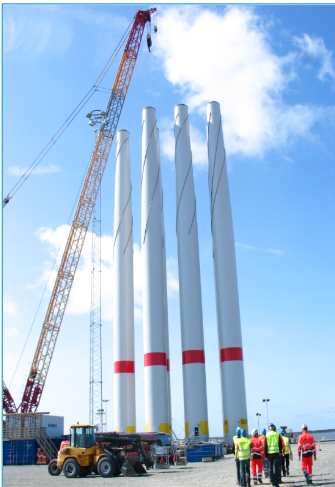
Figure 6.1.2-6. Towers assembled and ready for load-out.
