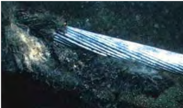
Figure 7.5: Fibre-optic cable with exterior sheathing recently damaged, presumably by fishing gear, to expose the bright steel armour, Cook Strait, New Zealand. Source: Transpower New Zealand and Seaworks.
