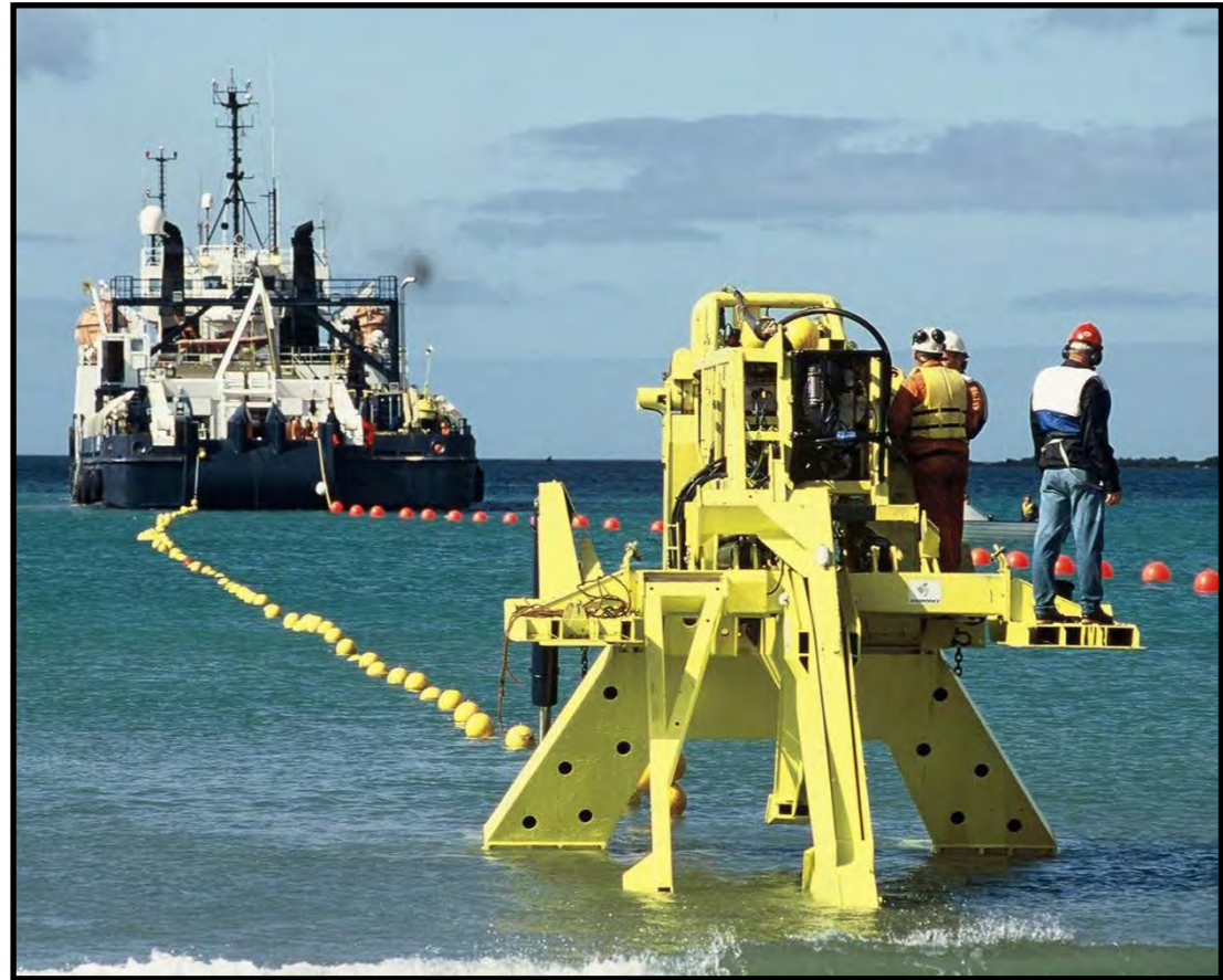
A plough being prepared to start the burial of a cable
