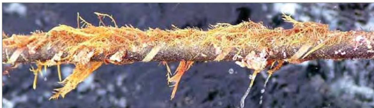
Figure 5.2: Surface-laid submarine cable, which has served as a substrate for the growth of epifauna. Source: Nigel Irvine.
