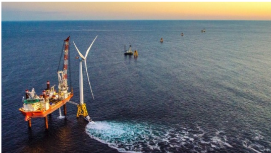
Block Island windfarm installation
