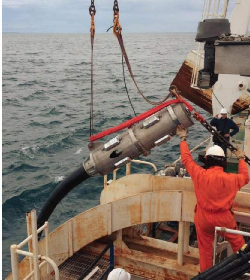
**Figure 2-7. Example of subsea connector (MacArtney’s GreenLink Inline Termination).**
