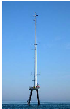
Source: Cape Wind Associates, LLC, 2012a Figure 3-2. Example of monopile mast meteorological tower
