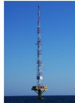
Source: GL Garrad Hassan, 2012 Figure 3-3. Example of a lattice mast meteorological tower with a monopile foundation
