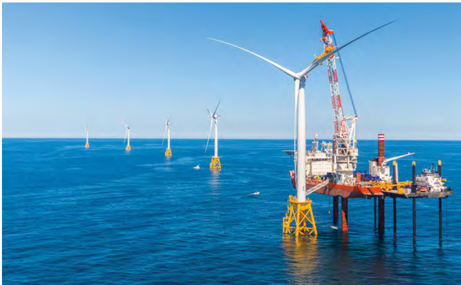
Installation of Deepwater Wind's Block Island Wind Farm, off Rhode Island. While offshore wind energy projects have not yet been developed in the Mid-Atlantic, several areas have been leased for that purpose. © DEEPWATER WIND
