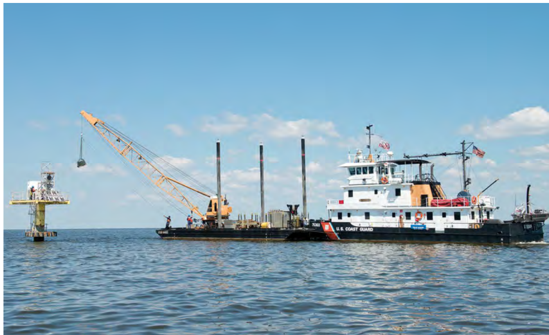
Crewmembers aboard Coast Guard Cutter Sledge use the ship's crane to lower a new transformer down to Craighill Entrance front range light Aug. 25, 2014. Crew members from Aids to Navigation Team Baltimore help guide the transformer onto the structure by use of the tag line.
