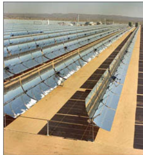
FIGURE 3 A Land-Based Parabolic Trough System (Source: NREL 2006b)
