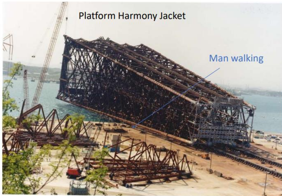
27 28 FIGURE 2-1 Platform Harmony Jacket Being Readied for Installation 29 (Photo credit: ExxonMobil).
