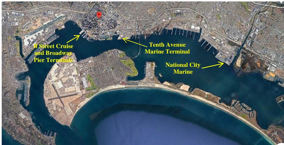
16 17 FIGURE 3.16-4 San Diego Harbor and the Port of San Diego (Source: Google 18 Earth 2021c). 19 20
