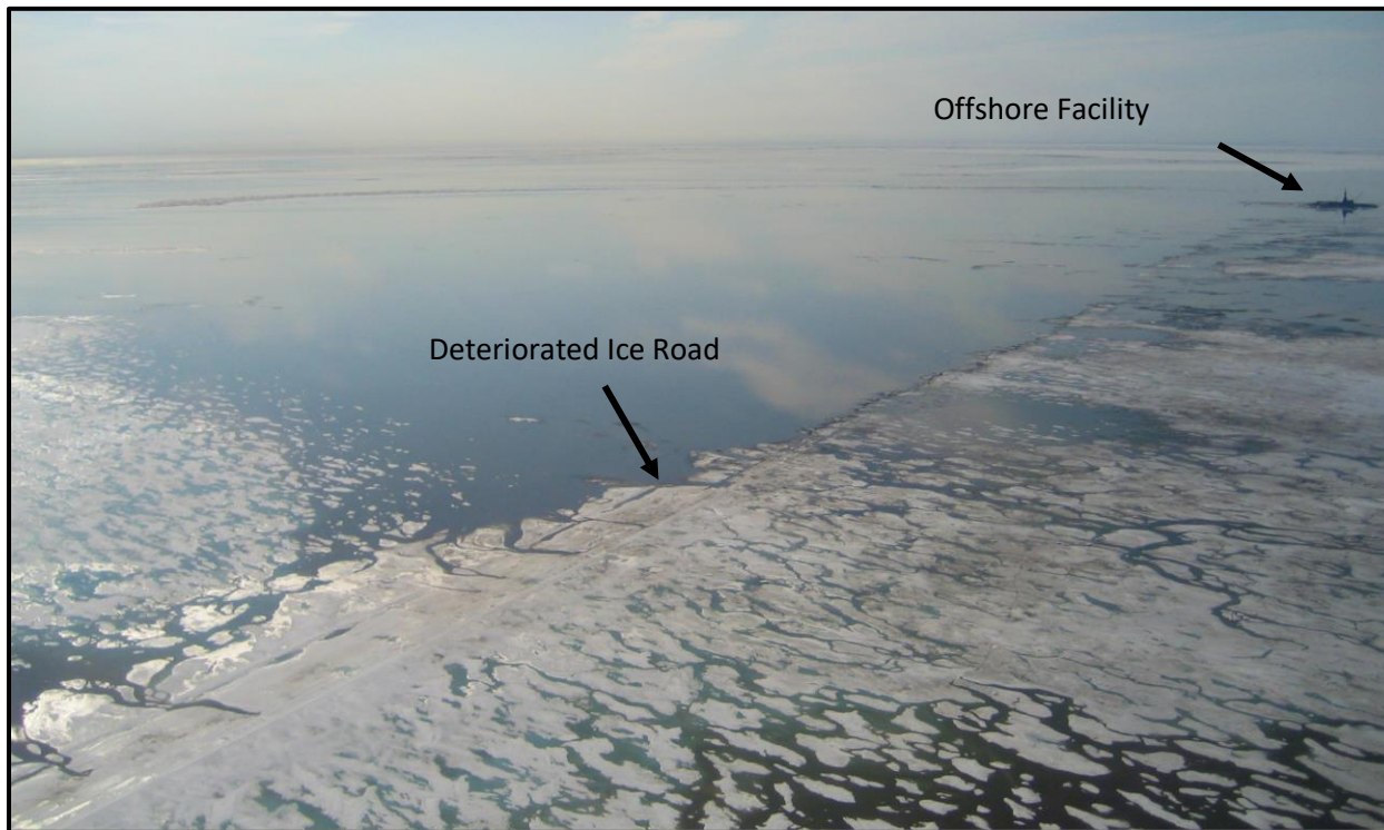
Figure 44. Damage to nearshore ice road due to flooding near the Colville River
