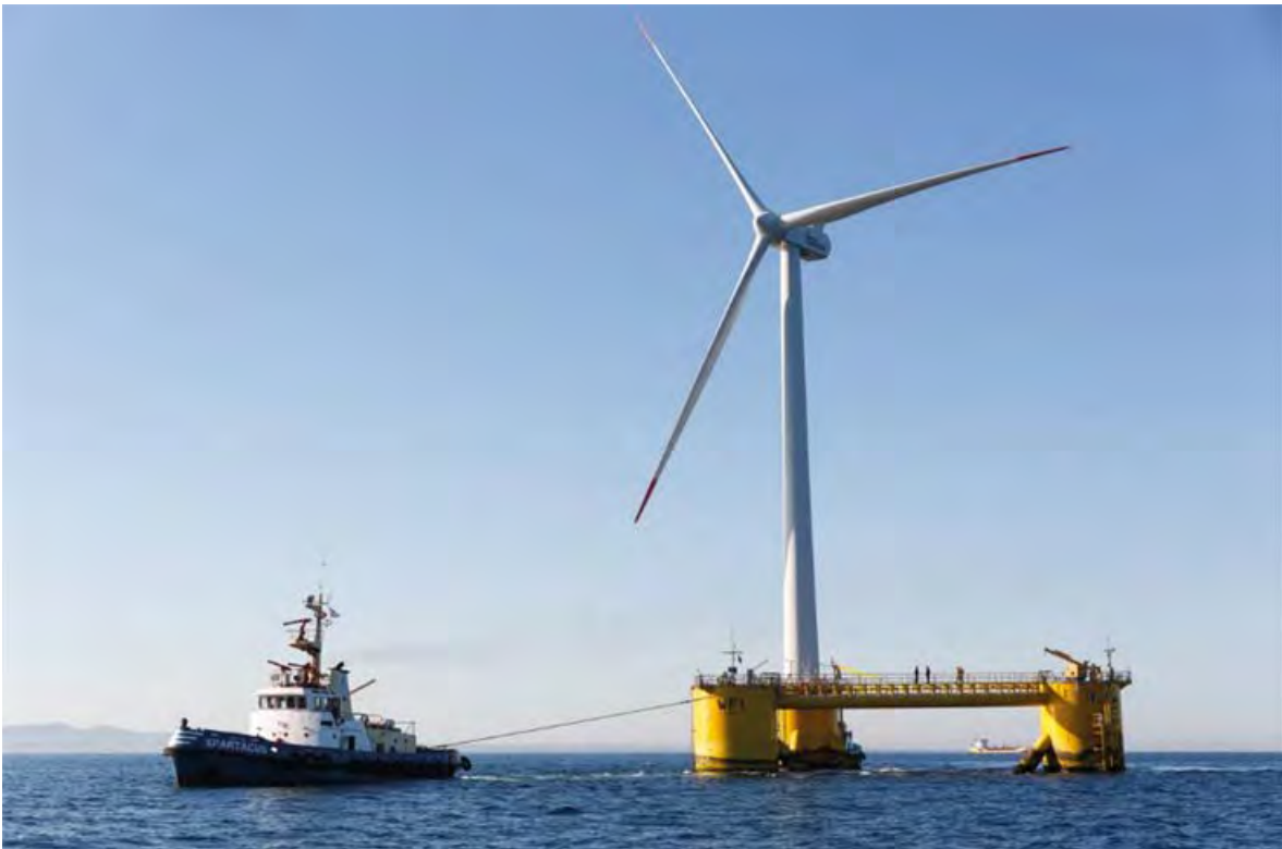
Figure ES-3. Principle Power semisubmersible with mounted turbine. Photo courtesy of Principle Power, Inc.
